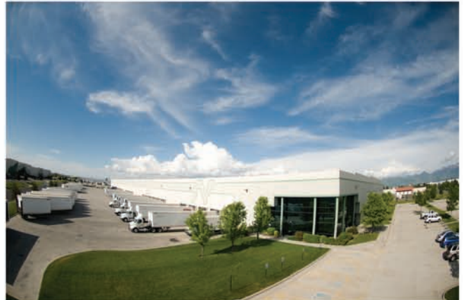
Aspen Warehouse in Salt Lake City, UT
